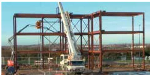
When the frame is complete, the concrete floors will be poured, paving the way for the erection of the outer cladding. This will allow work to begin on the interior of the building.
