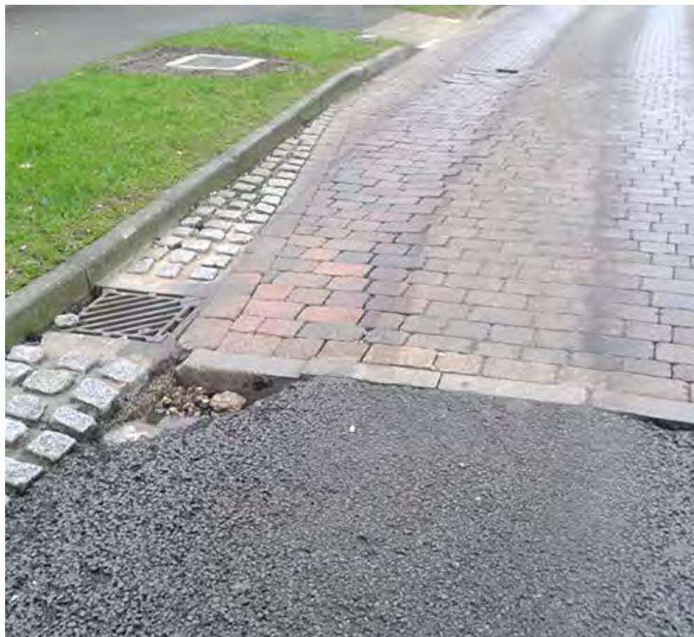
The carriageway is slowly subsiding and some blocks are missing. These could easily be hidden by standing water, and it seems likely that traffic movement could make it worse.
