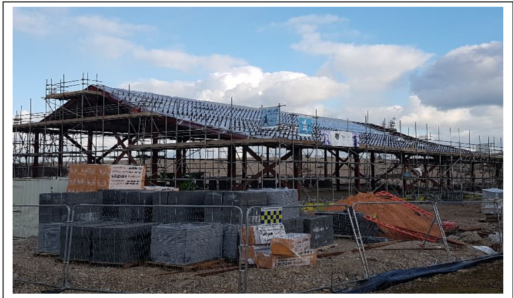
Full scaffolding in place to accommodate roof fixers and blocklayers
