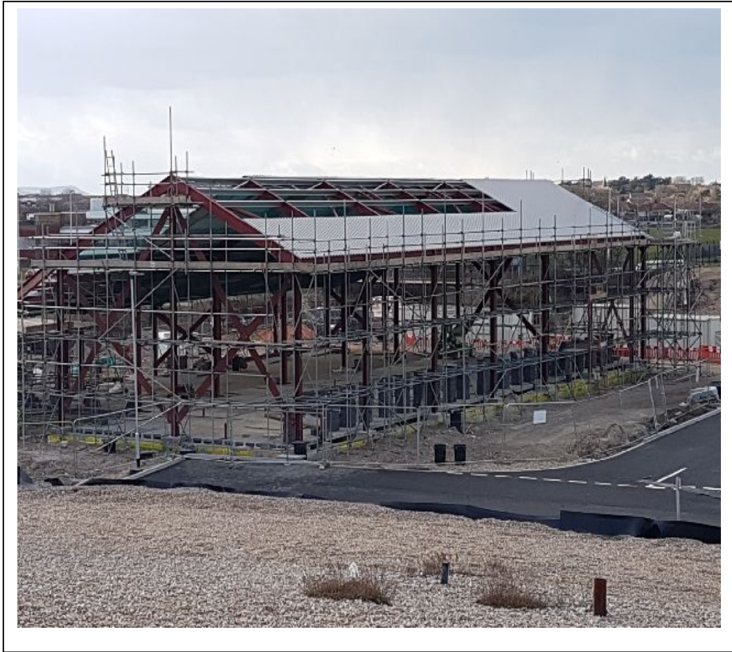
Full scaffolding in place to accommodate roof fixers and blocklayers
