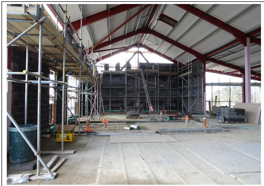
Blockwork is continuing, internal walls are underway
