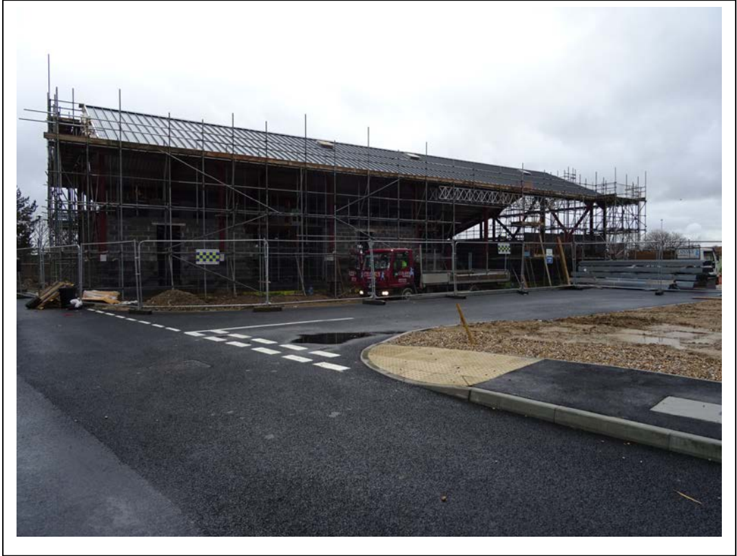
Blockwork is continuing, internal and external walls are underway
