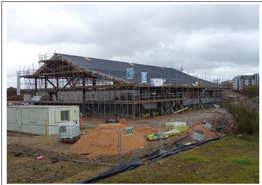
Blockwork is continuing, internal and external walls are underway
