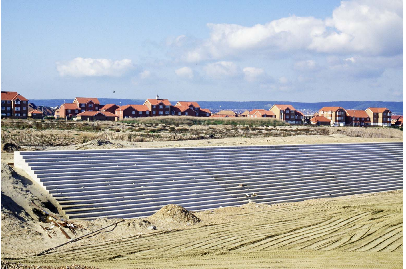
▲ Outer Harbour steps - only the top few steps are now visible.
