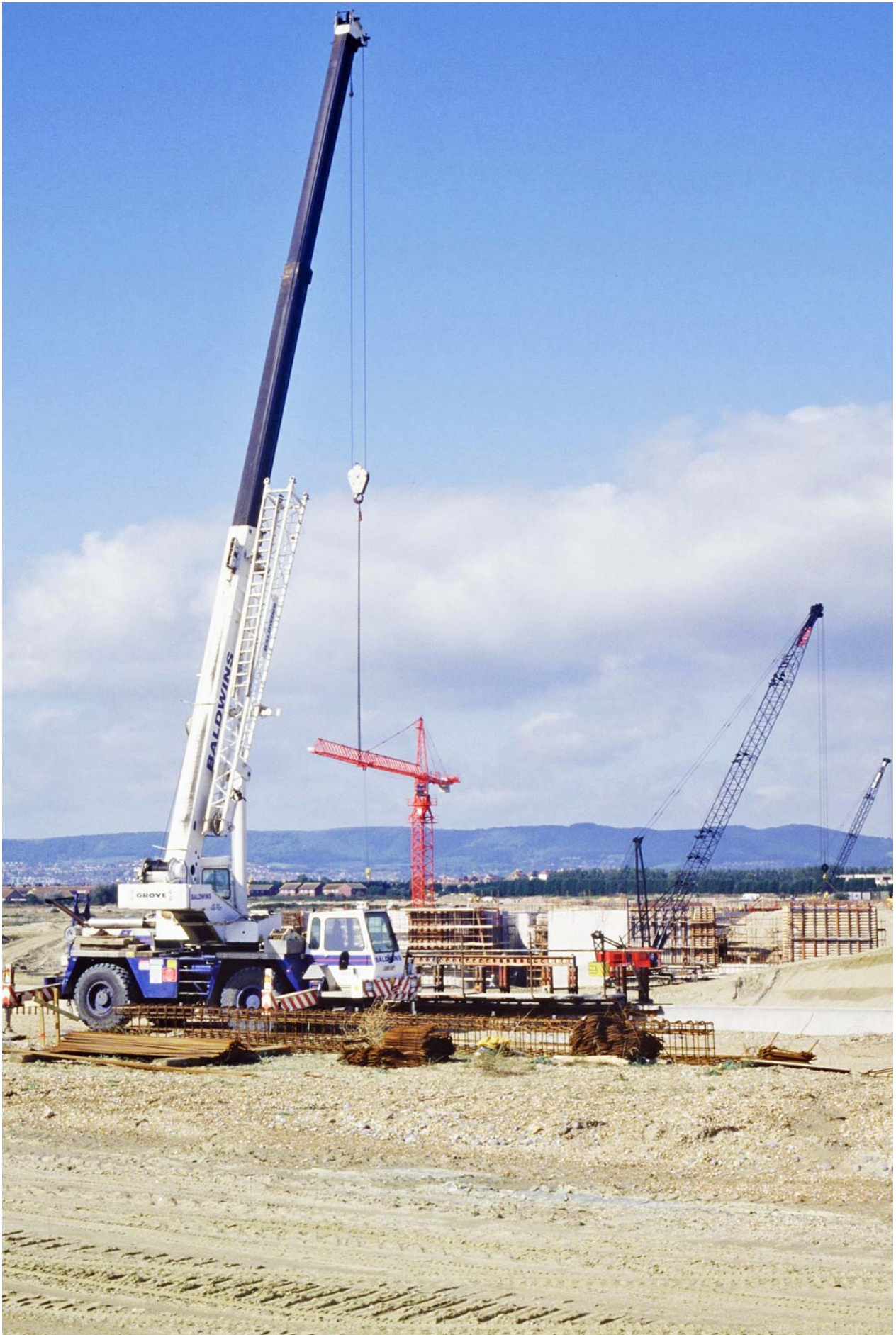
▲ Work on the Peninsular (foreground) and locks (background)
