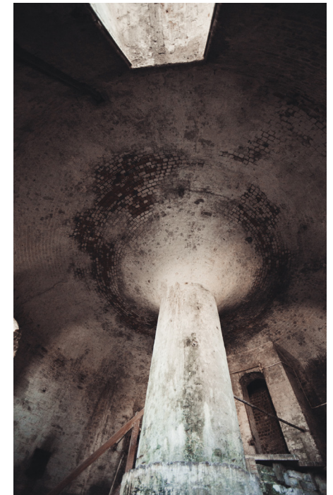
Internal view of Martello Tower 66
