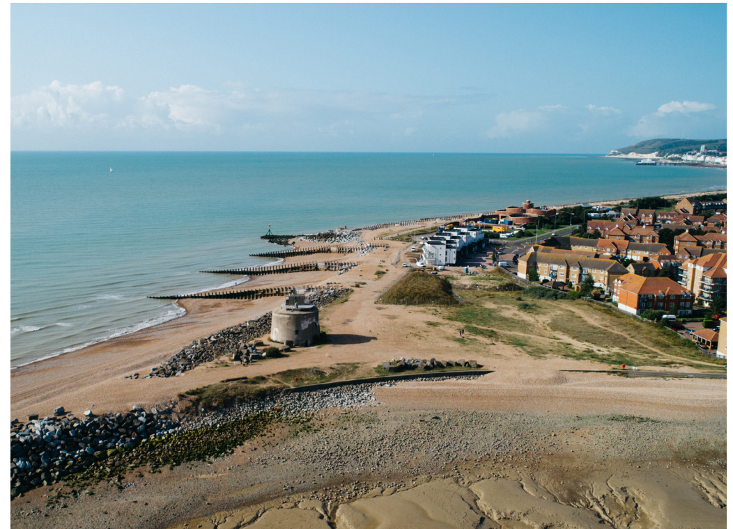
Aerial view of Martello Tower 66
