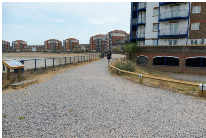
Loose gravel area used for crane access.
