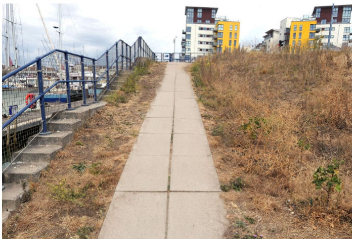
This steep, paved slope is now the only access up and down. It needs handrails.
